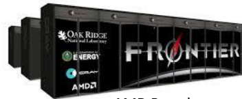
AMD Based (Up & running) 20 MW
